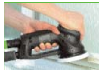
Coarse sanding of weatherboards.
